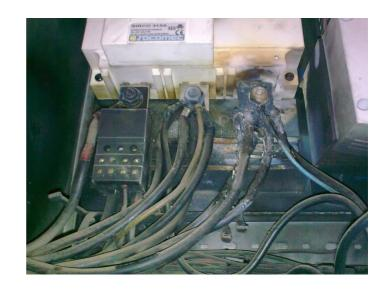
Thefollowing pictures were taken after we replaced the isolator, and damaged cables. We also fitted a bus bar arrangement so that the isolator lugs were no longer overloaded.
